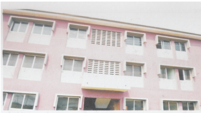
Egan Igando Housing Estate, Alimosho 684 units
