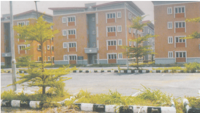
Igbogbo IIB Housing Estate, Igbogbo Ikorodu 360 units
